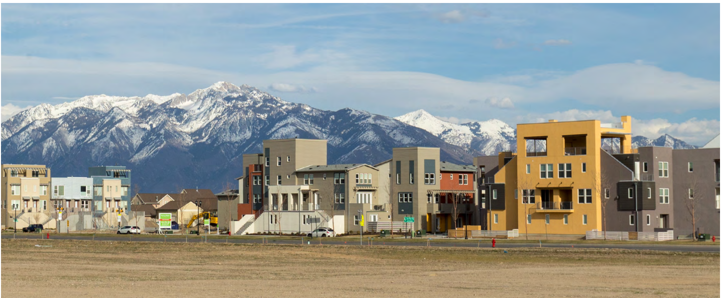
New construction provides an opportunity to build resilient communities in Utah.
