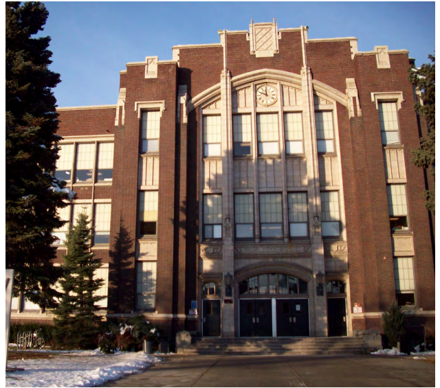
West High School is a URM school that was retrofitted in 1996.
